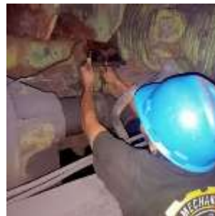
Gambar 9. Pengecekan Guide Wheel Manipulator Entry
